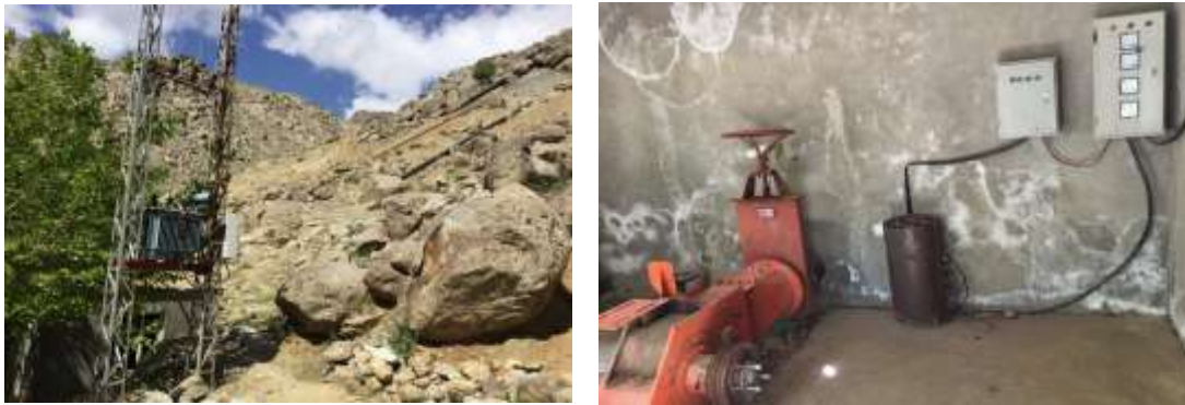
Figure 15 Pico-Hydro System in Sar-e-Nili, Daikundi
