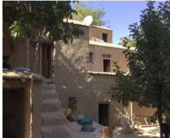
Figure 33 A television dish and solar panel crowning the rooftops
