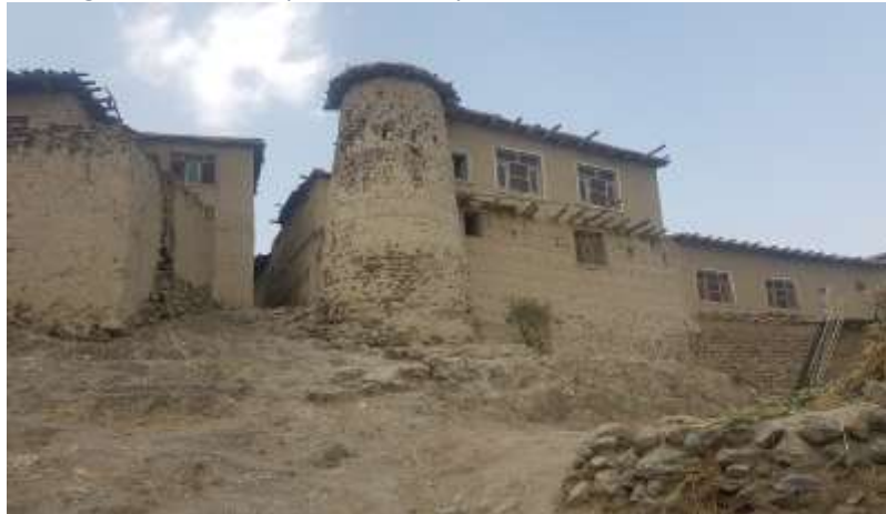
Figure 30 Powered by solar electricity - the house in Mondokhail, Paktia
