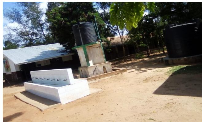
Picture 4 – Handwashing facilities in Mombasa with water but not soap
