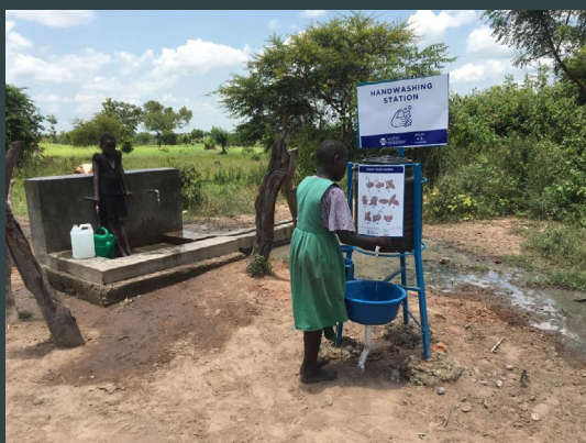
Hand washing facilities
