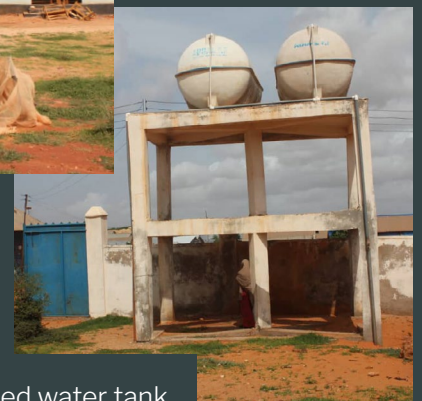
Elevated water tank
