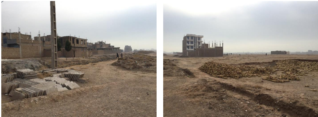
Photo 9 A panorama of construction in Talab-e-Ulia, Herat, where AVM lands were released by the HALO Trust
